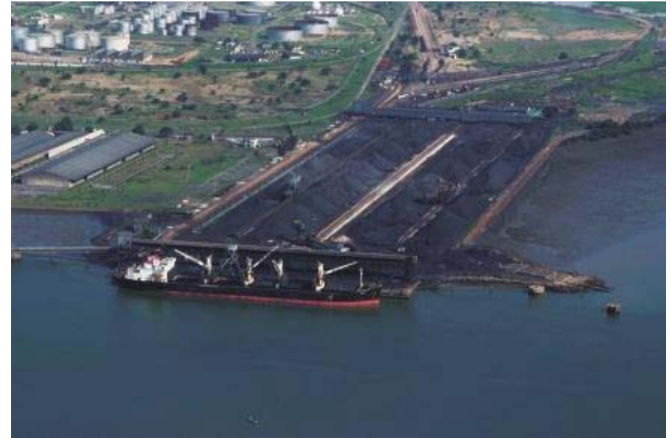
Matola Dry Bulk Terminal, Maputo (Mozambique)
